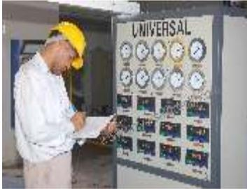
Instrument-control system, the window of the whole plant, could reflect all the information of the plant during its operation. A common instrument-control system is equipped with side by side cabinet and digital display together to reveal those parameters as pressure, temperature and flow rate. It is easy to operate, and the cost is relatively little.
