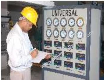
Instrument-control system, the window of the whole plant, could reflect all the information of the plant during its operation. A common instrument-control system is equipped with side by cabinet and digital display together to reveal those parameters as pressure, temperature and flow rate. It is easy to operate, and the cost is relatively little.
