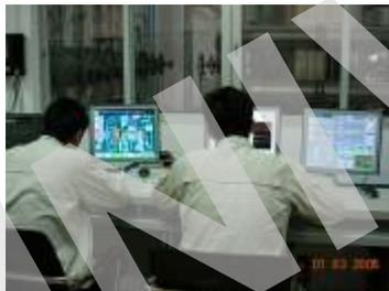
Centralized control system is equipped with PLC or DCS from Siemens for the function of display, operation, adjusting, memorizing, recording, alarming, interlock, start-up and shut down. In the computer, there are displays of main menu, process flow, parameter list, alarm and history trend. Network control of multi-computer is also achievable.
